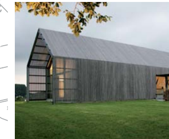
The Barn House, BURO2 Belgien
